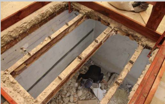
Breaking through to the lower level for an elevator shaft.
